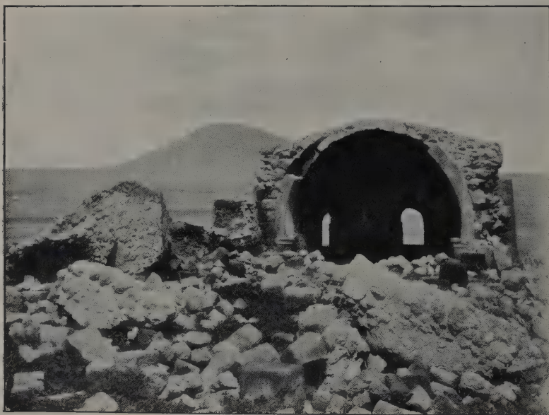
FIG. 35.—No. 6, interior of apse.
